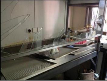
Figure 2. Glass shards remain in the sash frame after an explosion
