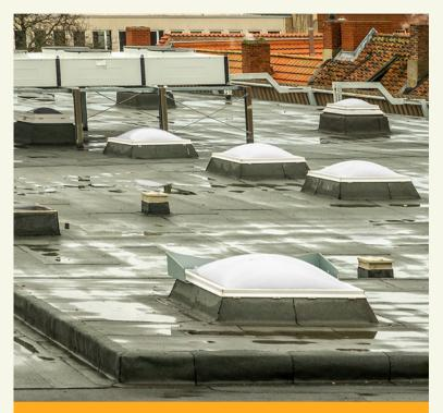
Cal/OSHA has a safety regulation that specifically addresses openings and skylights on a roof. If anyone is going to be within 6 feet of a skylight, one of these safety measures must be in place:
