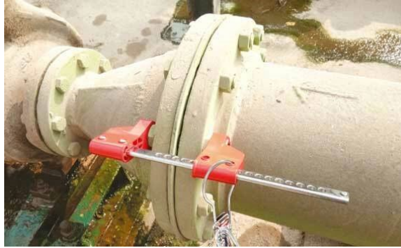
Blind Flange lockout on a pipe
