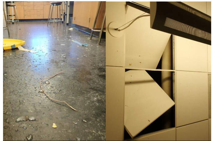
Glass and water were blown throughout the lab space. Enough force was generated to lift the tiles above the vessel.
